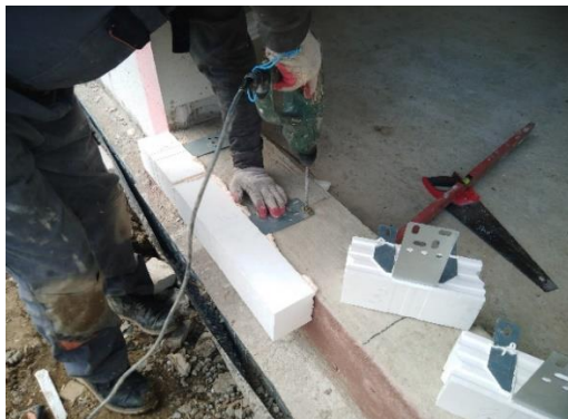
Photo 13 – Installation of CBM lower line
