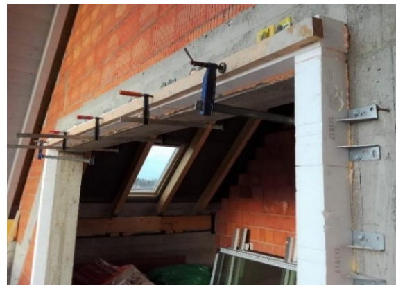
Photo 16 – Application of hand screws enhances and accelerates works
