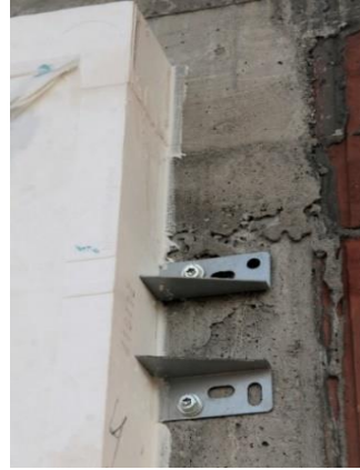
Photos 28; 29 – Skimming joints and CBM beams with a hybrid sealant in locations where water may accumulate and with an acryl on joints where water will not accumulate (e.g. flushing rain during setting )
