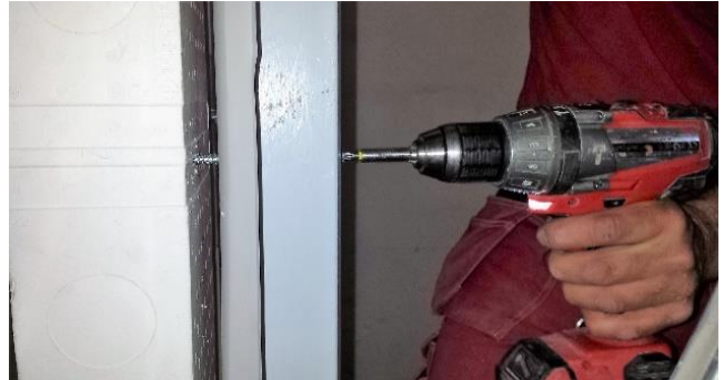
Photo 24 – Screwing in the window frames
