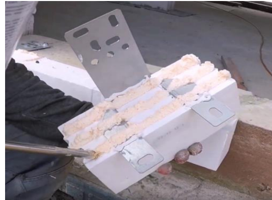
Photo 12 – Application of adhesive to PU EPS
