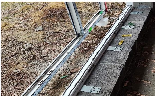
Photo 21 – Installation of the frame on the BP
