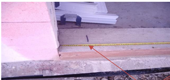
Photo 1 – Control measurement of the opening and arrangements of CBM beam axes
