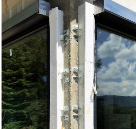
Photo 27- Installed nib (W)
