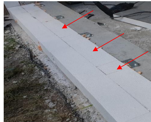
Photo 17 – Ground beams made of cut CBM beams with various thickness Photo 18 – Example of a ground beam for HST windows
