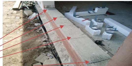
Photo 2 – anticipated location of installation axis
