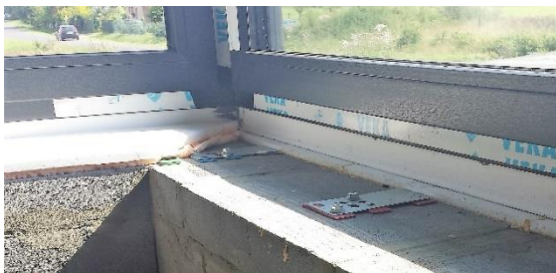
Photo 25 – Installation of internal window sills (PPW)
