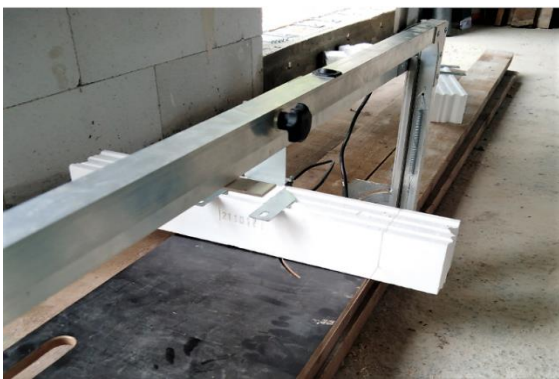
Photo 7 – Cutting CBM beams with a thermal string
