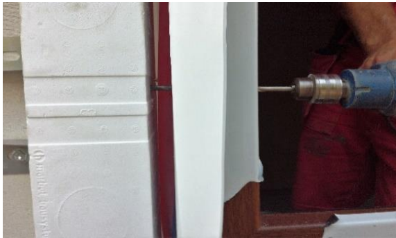
Photo 23 – Drilling holes in the brackets
