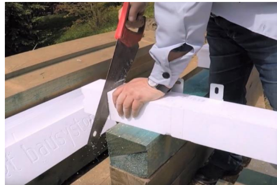
Photo 8 – Cutting CBM beams with a saw
