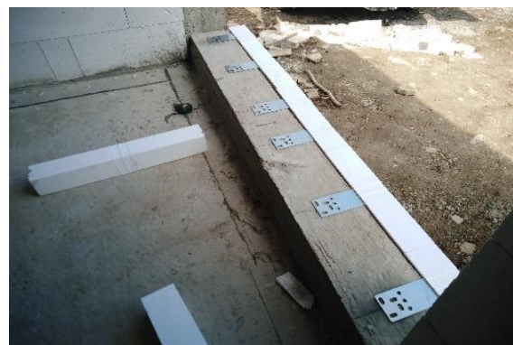
Photo 10 – Trial adjustment of re-cut beams
