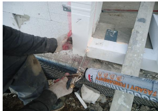
Photo 14 – Installation of CBM side line
