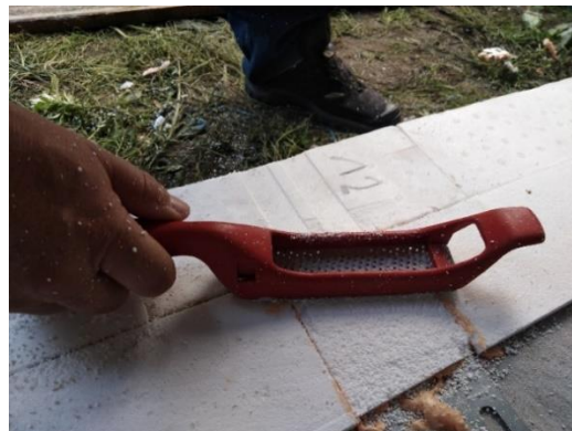
Photo 19 – Grinding with an oscillating grinder or a washboard
