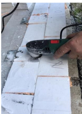
Photo 19 – Grinding with an oscillating grinder or a washboard
