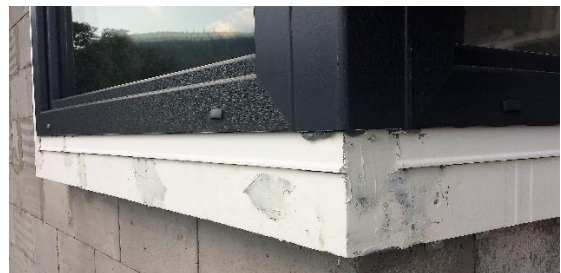
Photo 26 – Installation location for the base of the external window sill (PPZ)
