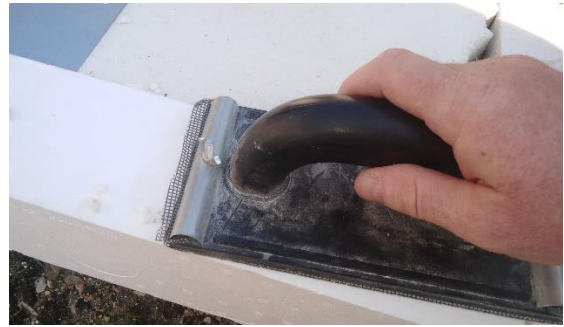
Photo 6 – Flattening and levelling of EPS surface for under-window beams with "EPS washboard" or other grinding tools
