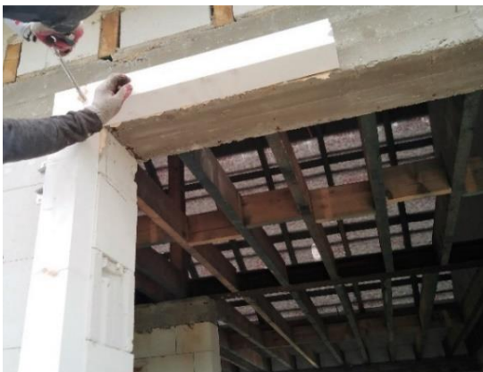
Photo 15 – Installation of CBM upper line
